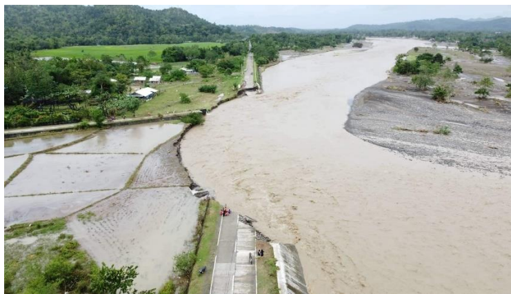
Fig. 1.18. Bridge collapsed in Antique, Western Visayas.
